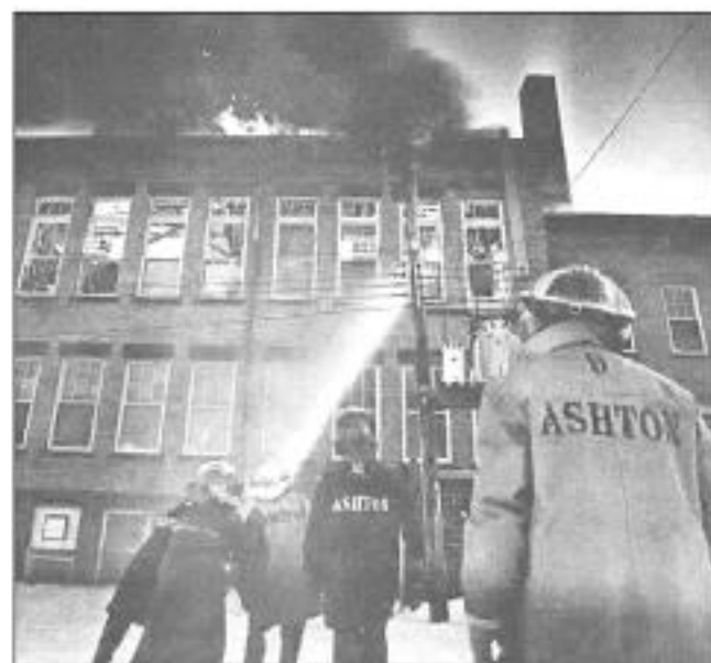
Ashton and Sibley firefighters battle a blaze at the Sibley Middle School on Thursday, Dec. 7, 1978. Five fire departments helped beat the flames before they could spread to newer wings of the building, but the central portion was considered a total loss. Heat tape installed on bell tower eaves to reduce ice buildup has been blamed by investigators looking into the fire which destroyed most of the 1902 portion of the middle school.
