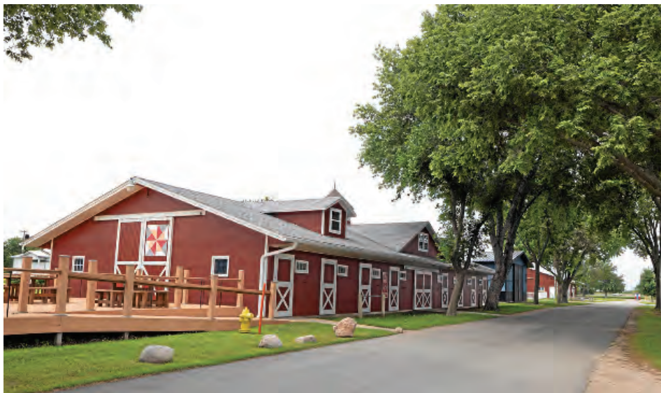
The horse barn which was repainted last year is shown as workers prepare the various buildings for the Clay County Fair.
