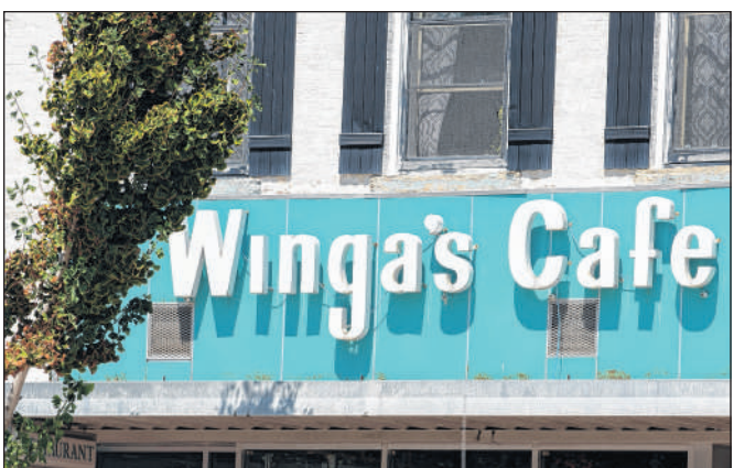
The old Winga's Cafe sign sits on top of the building that Isabella and Edward Santoro are renovating to turn into a diner in Washington.
