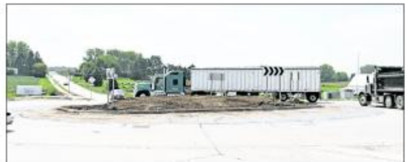
The Iowa Department of Transportation specifically engineered Orange City's roundabout to fit large trucks that use Highway 10. Photo by Mikaela Mackey
