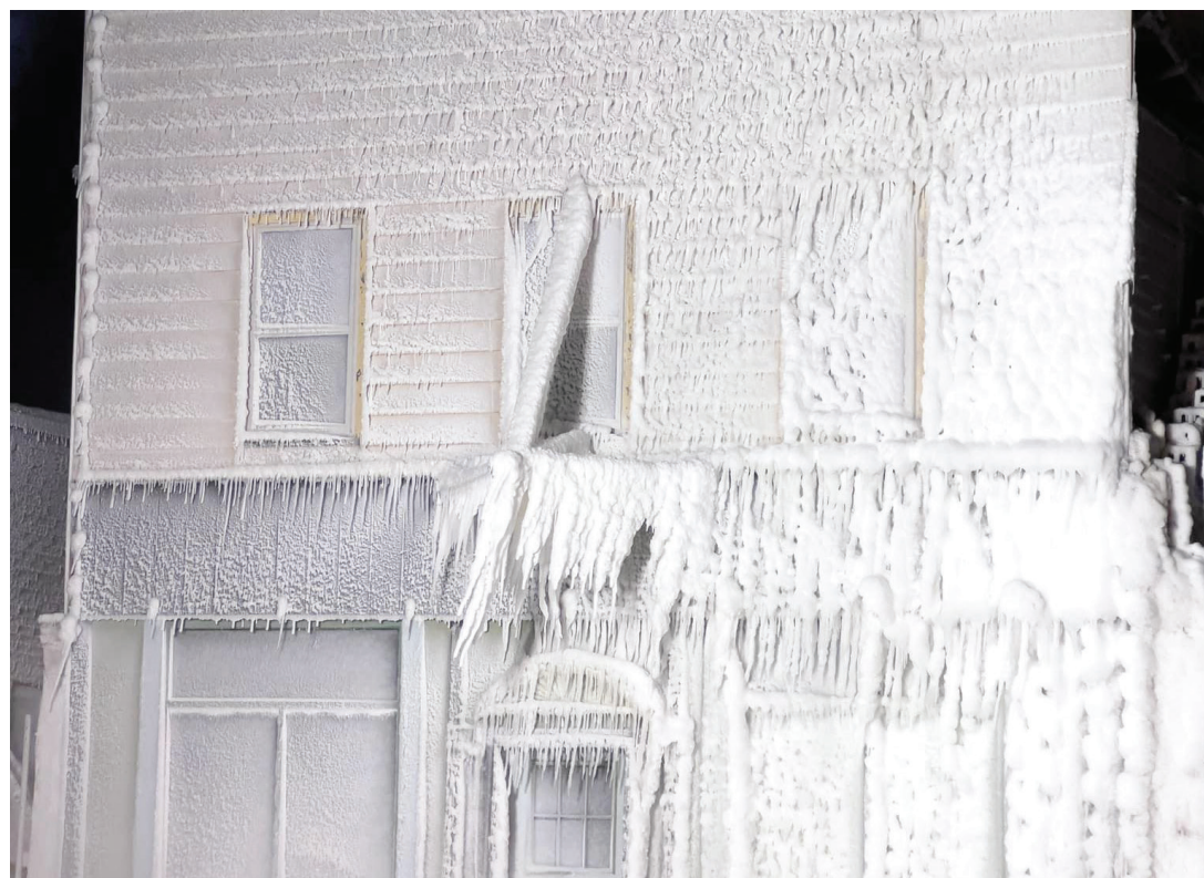
Frozen water and snow coats the exterior of a building in Spring Grove, Minnesota Thursday evening. Photo by Rick Aske
