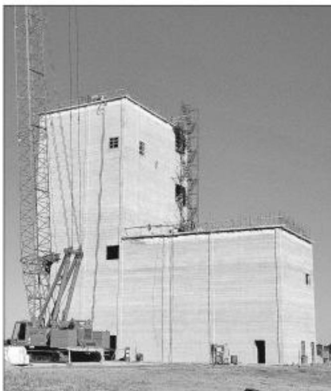
The Kent Feed Mill and Grain Science Complex will be a world-class, state-of-the-art facility used by faculty and staff to prepare students and train ag industry professionals. Photo submitted
