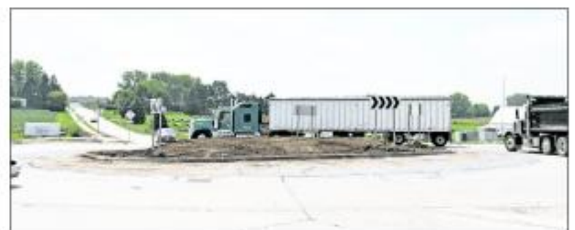
The Iowa Department of Transportation specifically engineered Orange City's roundabout to fit large trucks that use Highway 10. Photo by Mikaela Mackey
