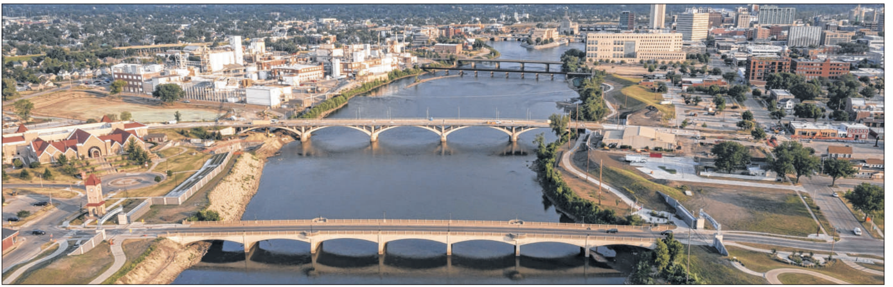
Flood gates, berms and flood walls are visible on both sides of the Cedar River near the 16th Avenue Bridge (foreground). (Nick Rohlman/The Gazette)
