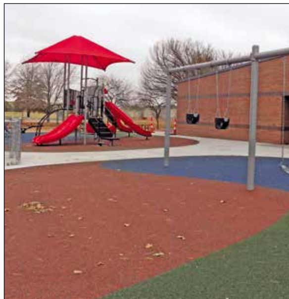
The new pre-K playground, completed this month.
