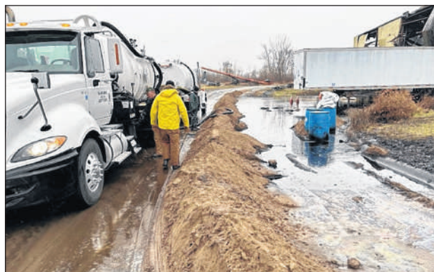
EcoSource employees use vacuum trucks to collect contaminated water in early December 2022 around the C6-Zero site in Marengo. Blue drums sitting in water are firefighting foam brought to the blaze. (Photo from EcoSource Environmental Assessment Plan)
