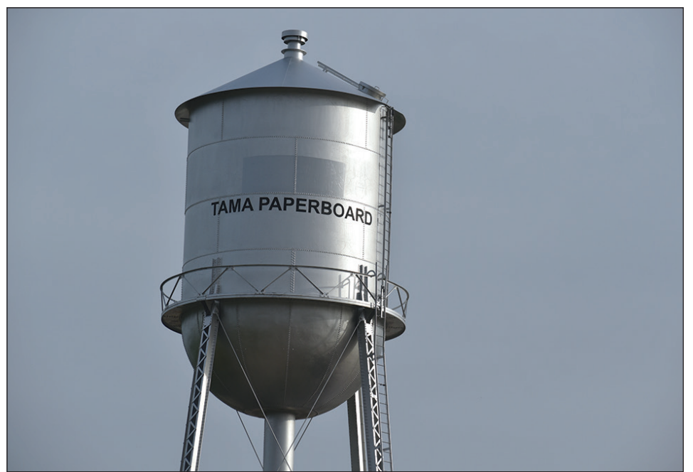
A close-up of the water tower at Tama Paperboard, which will be closing its doors on June 2.
