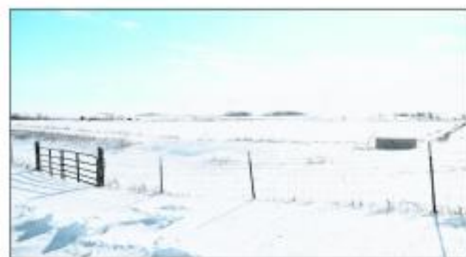
This iced-over wastewater treatment lagoon owned by Primghar is one of three that will be consolidated into a single unit thanks to $500,000 from a state assistance program grant allocated to water quality infrastructure upgrades. Photo by Eric Harrold
