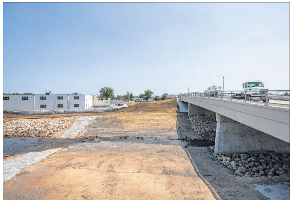
A truck May 23 drives over the Shaver Road Bridge in Cedar Rapids. Instead of installing a floodgate on the road, the city configured it as a raised bridge. That way, the major truck route can remain open as floodwater rushes underneath. (Savannah Blake/The Gazette)
