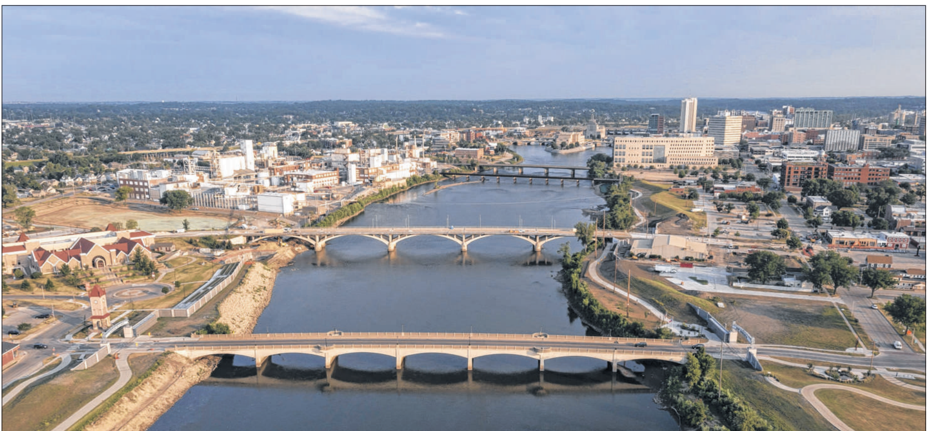
Flood gates, berms and flood walls are visible Thursday on both sides of the Cedar River near the 16th Avenue Bridge (foreground). (Nick Rohlman/The Gazette)
