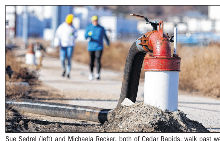
Sue Sedrel (left) and Michaela Recker, both of Cedar Rapids, walk past wells heads along the Cedar Lake Trail on March 2 in northeast Cedar Rapids. The wells were drawing water out of the lake in preparation for a flood protection levee. Work will begin on the ConnectCR Trail and amenities once the levee is complete. (Jim Slosiarek/The Gazette)
