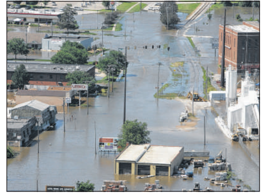
Part of First Avenue in Coralville remains under water June 16, 2008.
