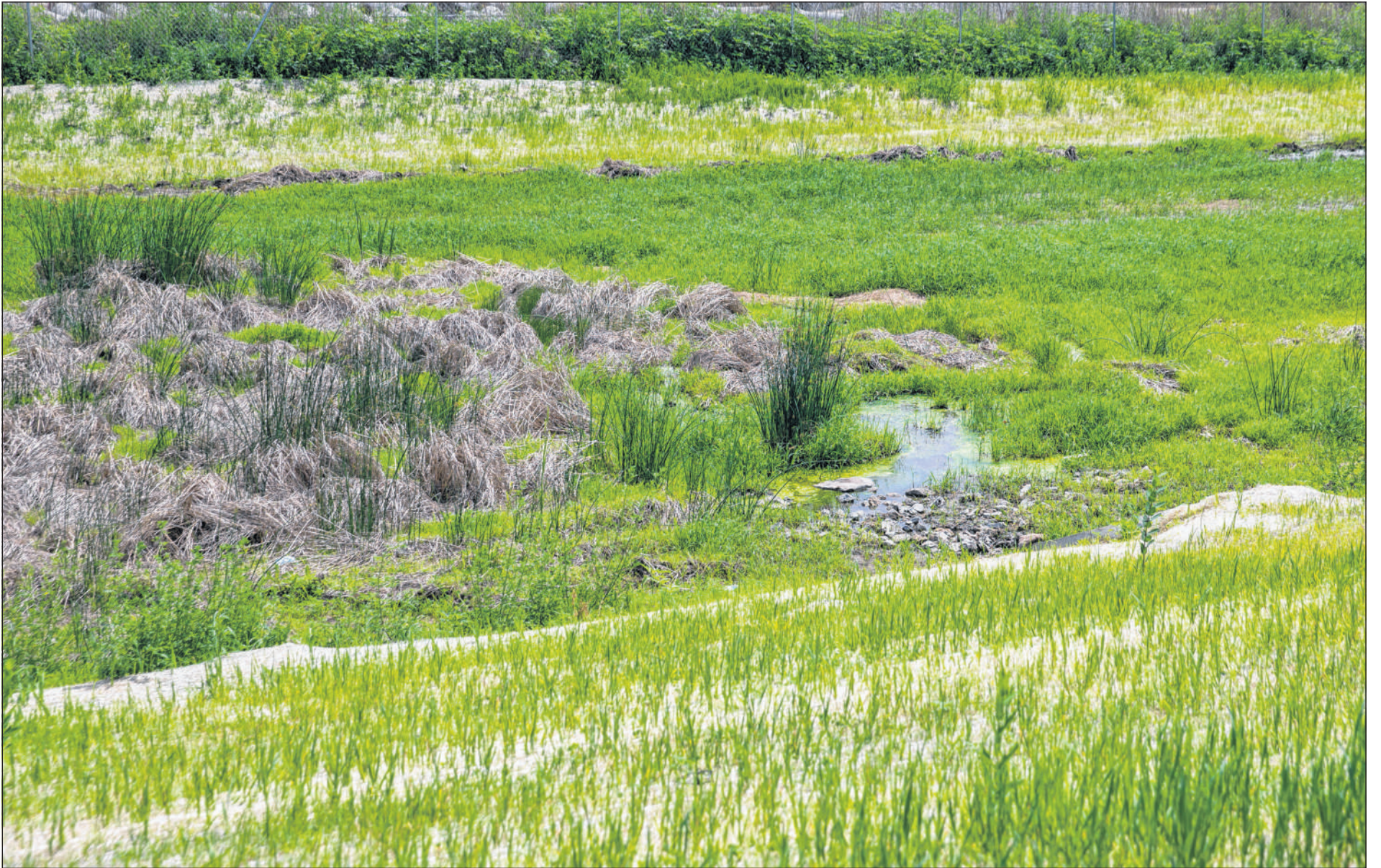
A bioretention cell sits just outside the new Cedar Falls High School in Cedar Falls. The space will utilize water runoff to water future plants and natural wildlife. (Savannah Blake/The Gazette)
