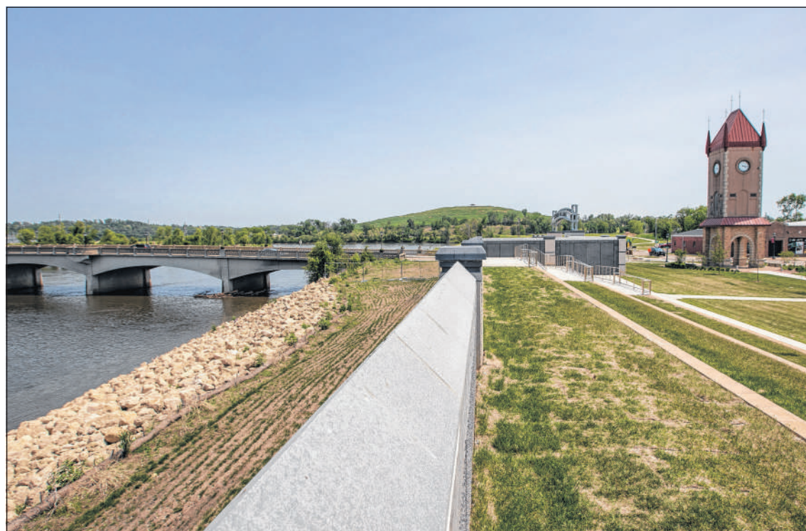
A flood wall hugs the Cedar River near 16th Avenue SW in Czech Village in Cedar Rapids. The concrete wall stretches 13 feet high, extending to the 16th Avenue Bridge. There, floodgates can be rolled into place to protect Czech Village from river flooding. (Savannah Blake/The Gazette)
