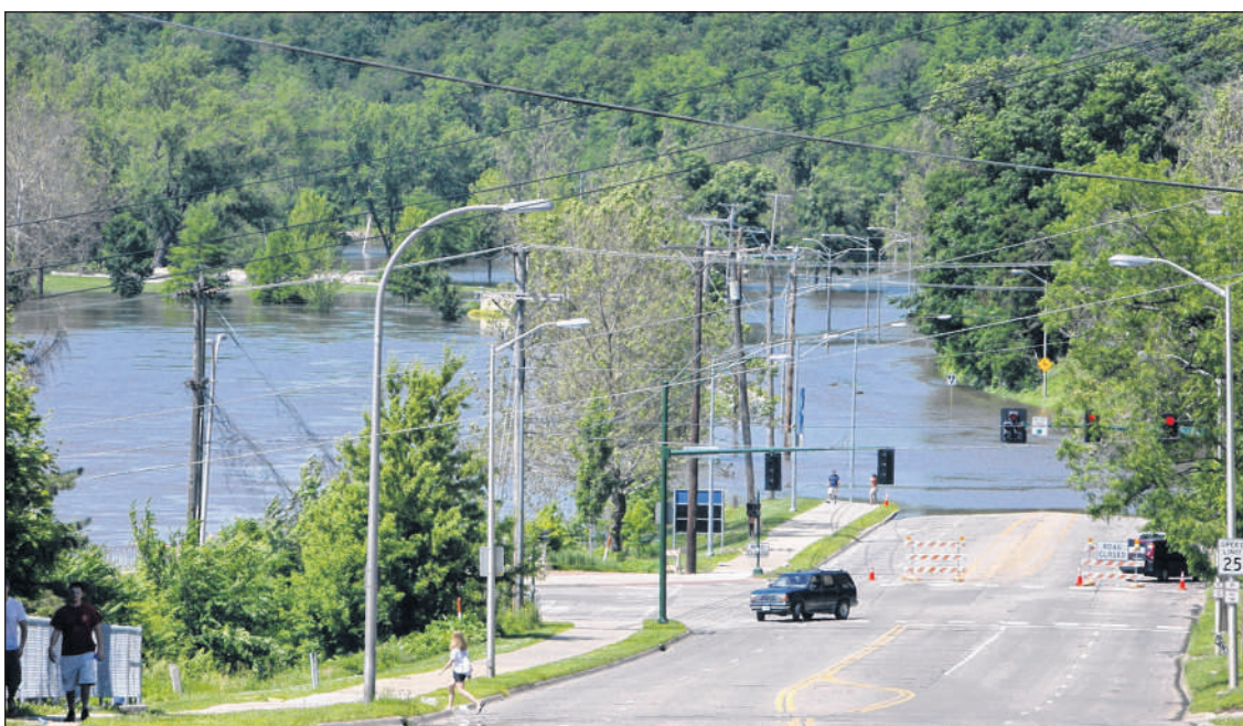
On June 10, 2008, floodwater covers Dubuque Street near the Park Road Bridge in Iowa City. Five days later, the Iowa River crested in Iowa City at a record 31.53 feet. (The Gazette)
