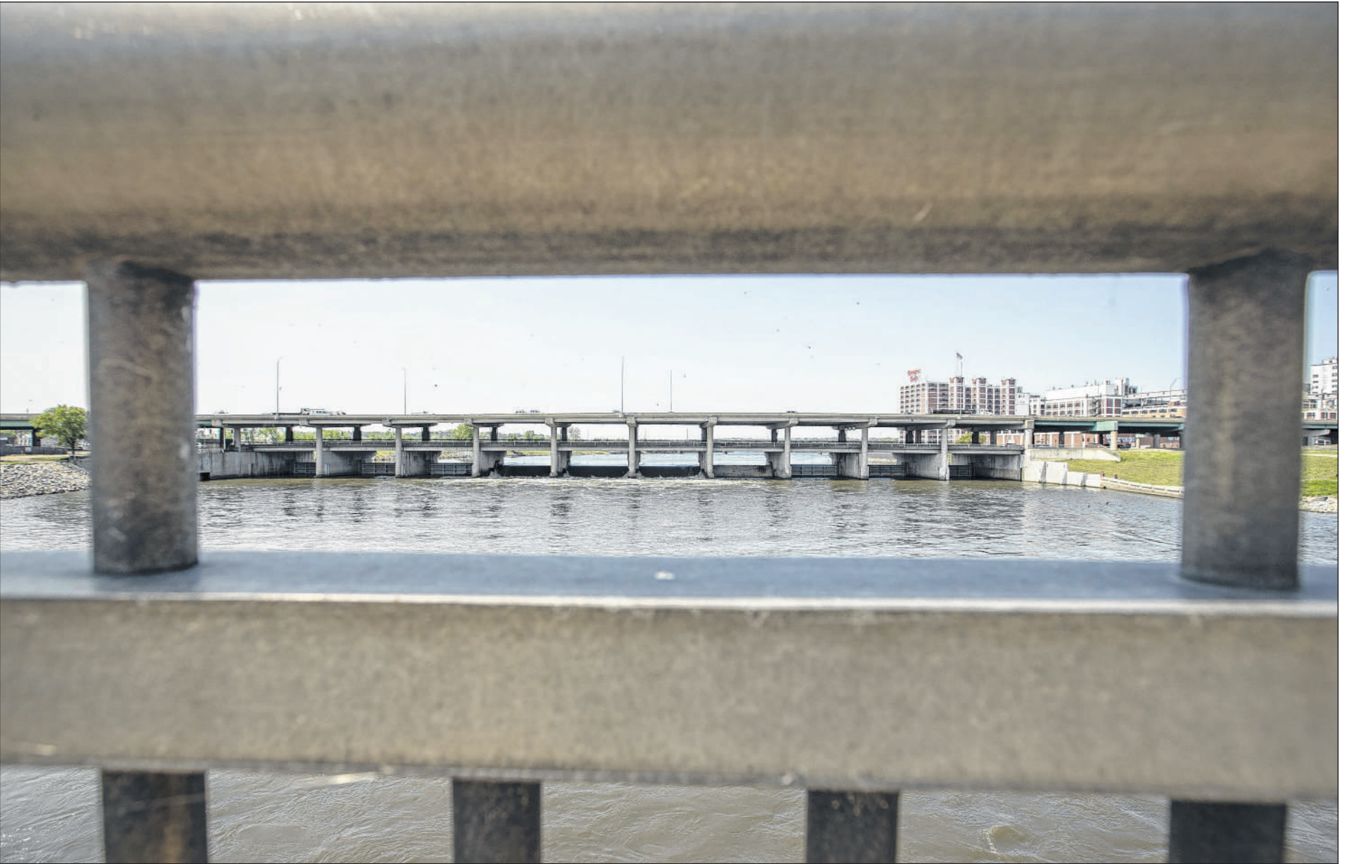
Traffic drives May 23 across the 5-in-1 Dam in Cedar Rapids, where flood walls and levees will line both banks of the Cedar River. (Savannah Blake/The Gazette)
