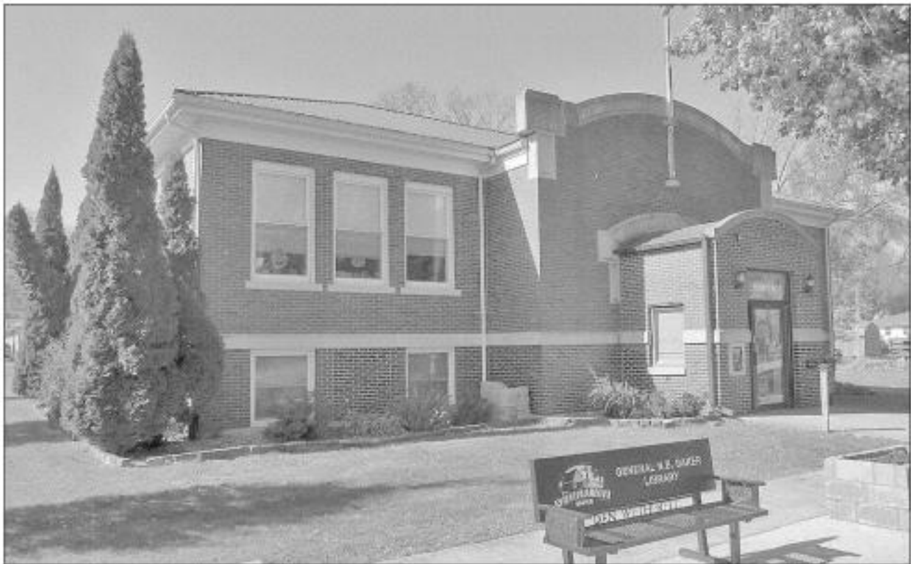
Repairs to the Gen. N.B. Baker Library are under consideration by the Sutherland City Council as the structure's foundation is cracking. The city decided to get quotes on projects costs after discussing the issue on Monday, Feb. 6. Photo submitted
