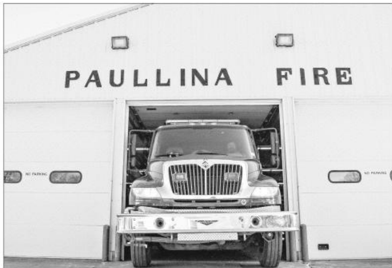
It's a tight squeeze just about everywhere at the Paullina Fire Department including equipment parking, and replacing the station is being pursued. Funding from the Paullina Emergency Services Golf Tournament will help out. Photo by Elijah Helton
