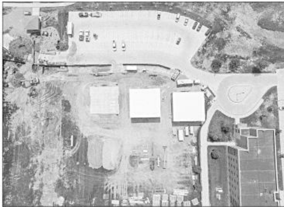
Dordt University in Sioux Center underwent several renovation and construction projects this summer to secure additional classroom space, housing and parking options. Photo submitted
