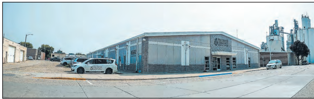
Promise Community Health Center in Sioux Center hopes to break ground in August on a $5.1 million expansion on the east side of its 33 Fourth St. N. building. Project plans call for constructing a 10,000-square-foot, two-story addition on a gravel portion of property owned by Promise that now serves as staff parking. Photo by Renee Wielenga
