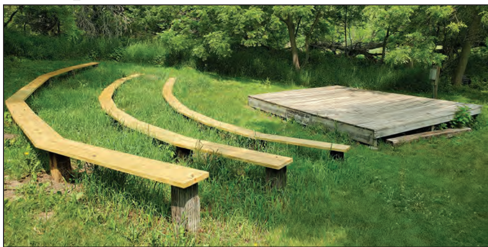
The amphitheater located in the Dunham Prairie Preserve, along the Ron Wilmot Walking Trail, has a fresh new look -- compliments of Akron Parks & Recreation Board Member Paul Bernard who replaced and varnished the seating.
