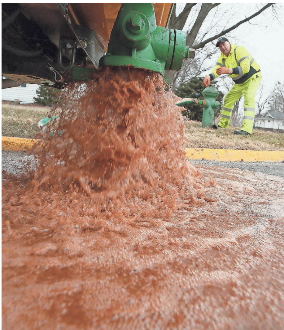
Ames city employee Jason Bohning flushes the hydrant.
