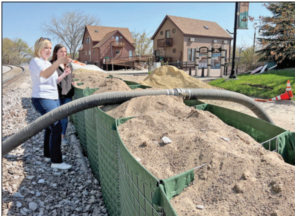
Rep. Ashley Hinson surveyed areas impacted by flooding during a visit to Clayton County on May 4. Here, she and Clayton County Emergency Management Coordinator Sarah Moser look at the HESCO barriers erected along the Marquette riverfront. (Photo by Audrey Posten)
