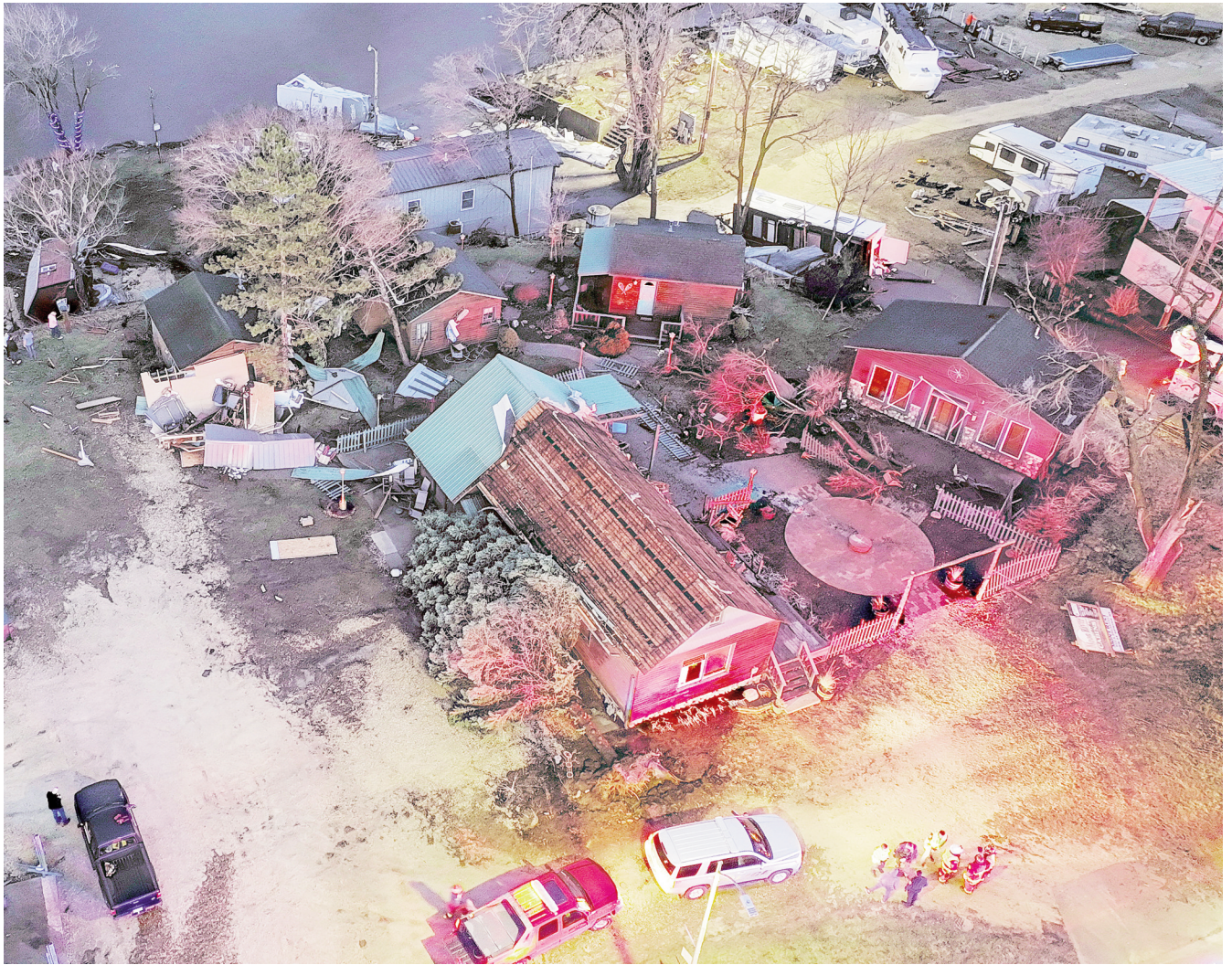
DAMAGE TO MOON RIVER CABINS is shown here just after the storm passed through Bellevue last Friday night. (photo courtesy of M.L. Beauchamp)
