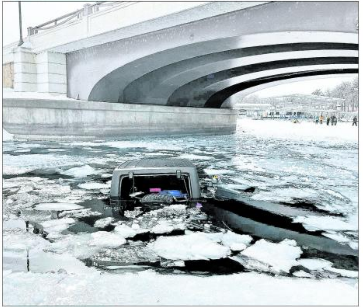
A Jeep owned by Thomas Lee of Milford sits partially submerged under the Highway 71 bridge that spans the channel separating East Lake Okoboji from West Lake Okoboji. Lee and his dog, Cooper, were rescued. Photo submitted
