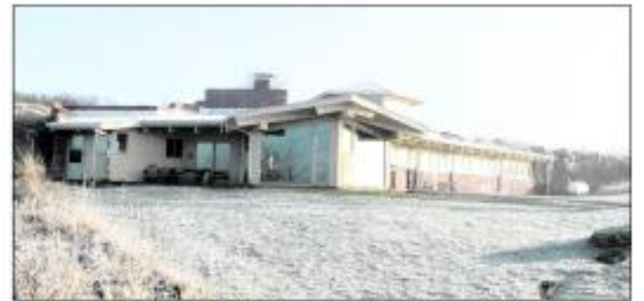
The Manfred House at Blue Mounds State Park outside of Luverne, MN, still stands. It was built by Doon native and writer Fred Manfred and his daughter wants the house restored. Photo by Elijah Helton
